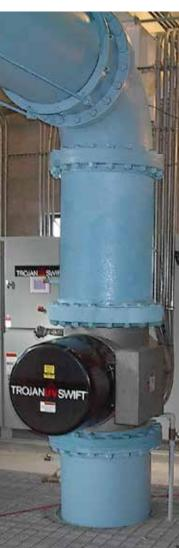
Compact footprint enables the integration of the TrojanUVSwift into restrictive pipe galleries – reducing installation costs and eliminating the need for larger buildings or additions.
