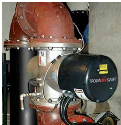
*Compact footprint enables the integration of the TrojanUVSwift into restrictive pipe galleries – reducing installation costs and eliminating the need for larger buildings or additions.*
