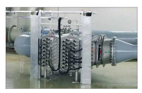
The chamber has been designed for delivery of high UV doses in an extremely compact footprint (40% to 50% that of other high efficiency UV-oxidation systems).
